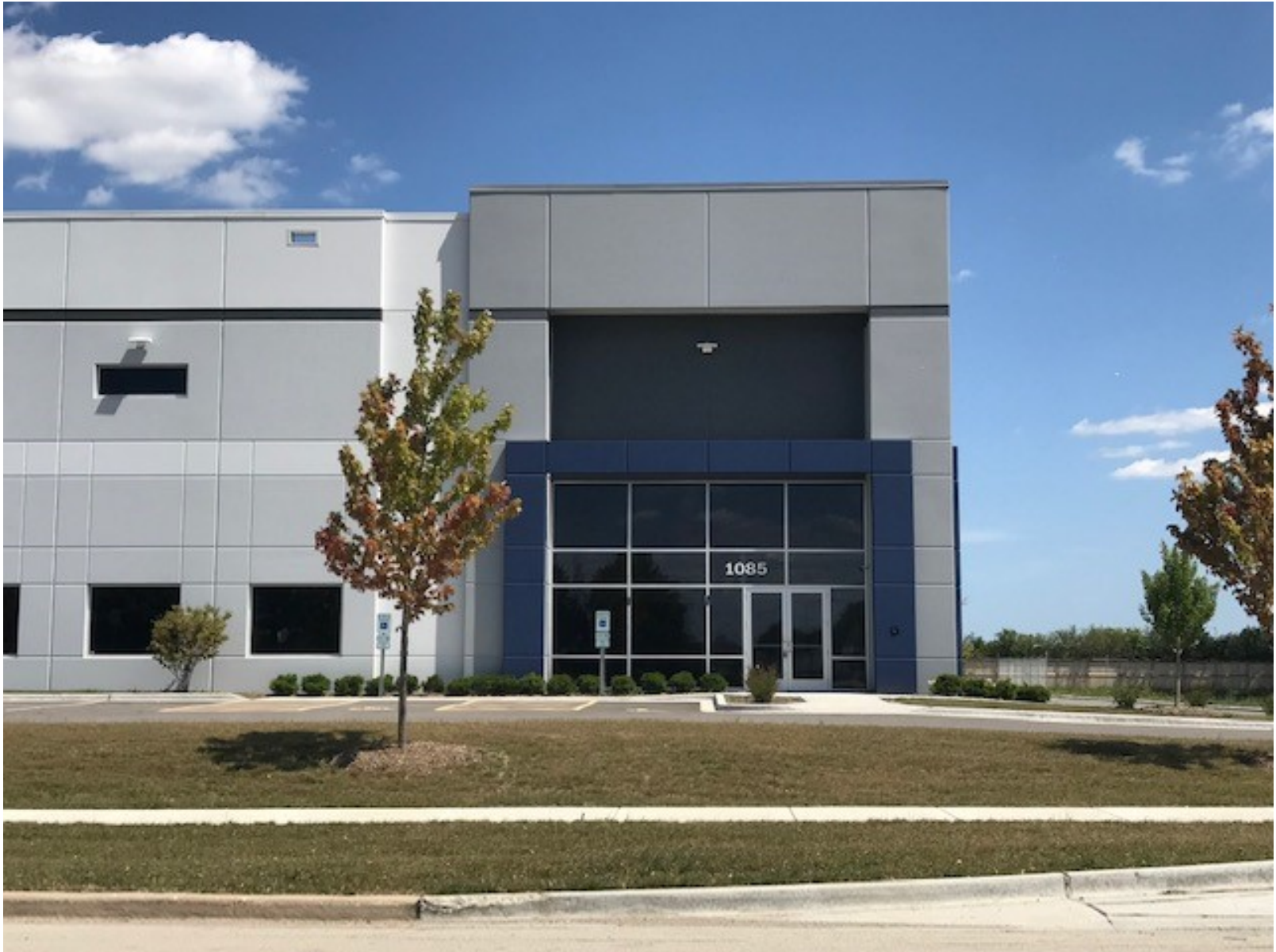
Existing conditions of front elevation (looking east)
