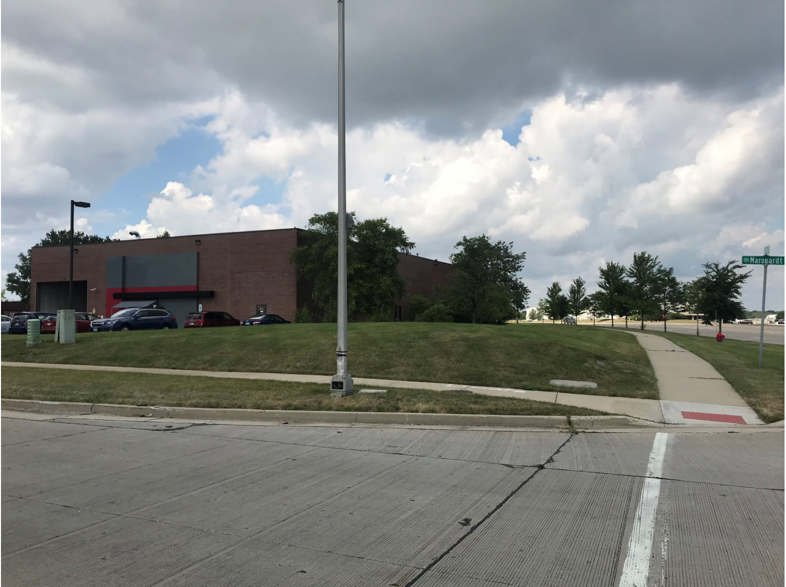
Existing conditions of front elevation (looking north)
