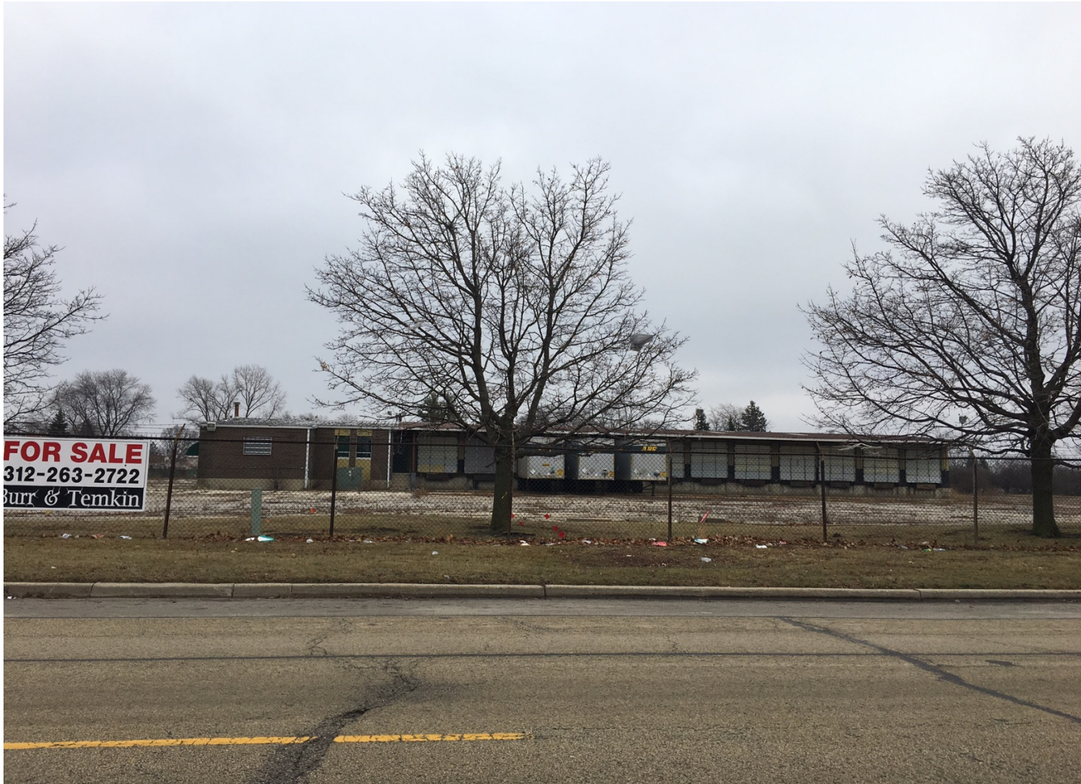
Existing conditions of subject property (looking east)
