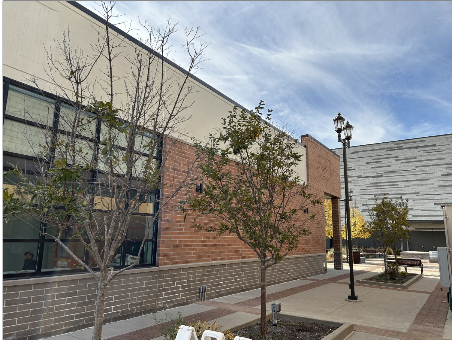
North side of the building, location for wall sign extending above roofline.
