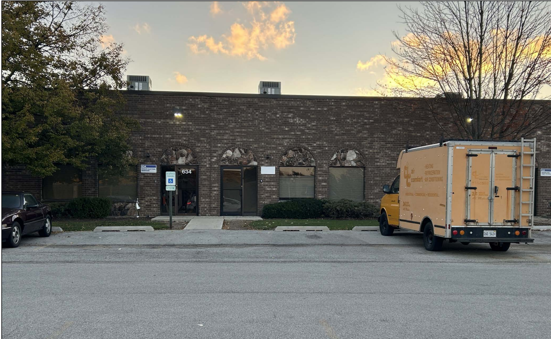
Photo of the Front of the Business Facing East from the Parking Lot.
