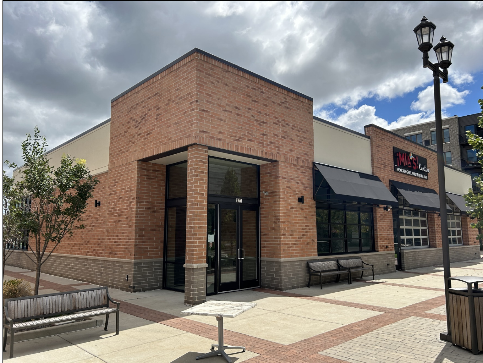
Southwest corner of building, location for canopy sign.
