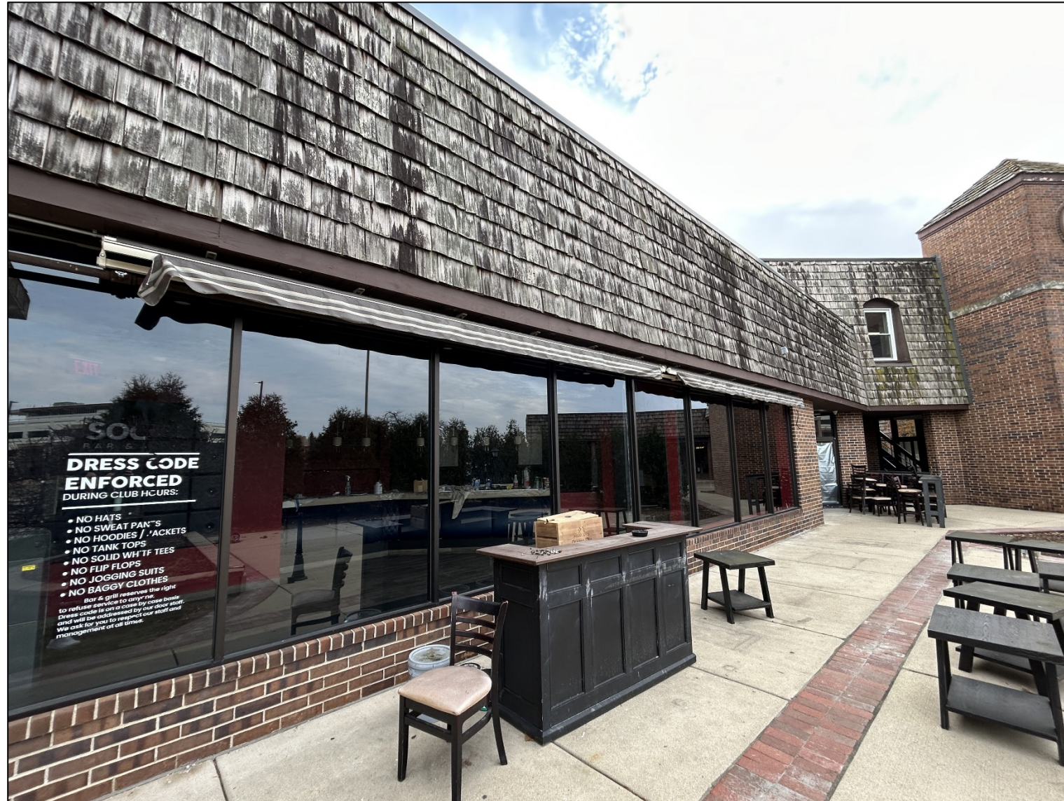
Photo of fabric awnings that must be removed.
