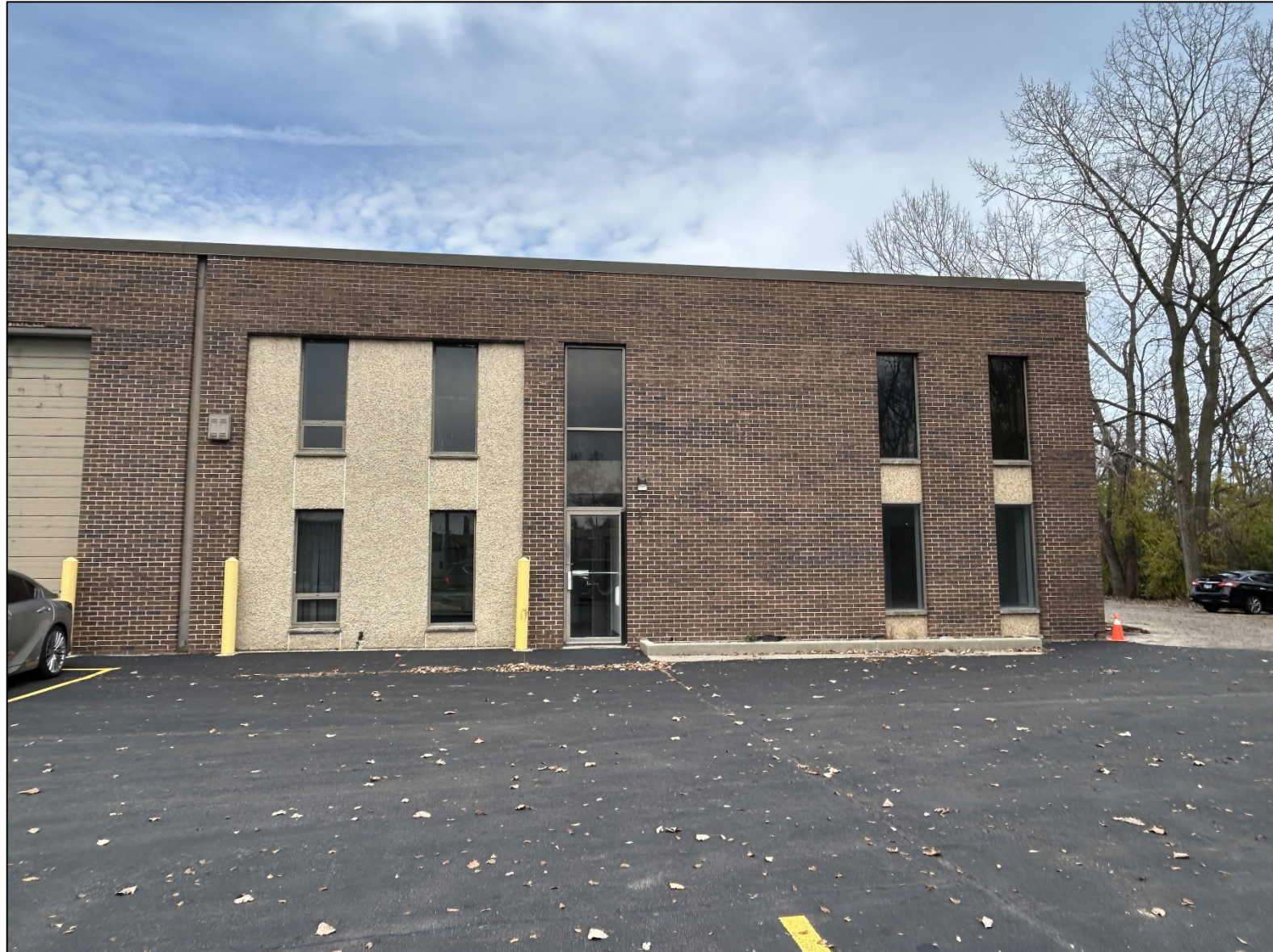
Proposed Business Entrance, East Side of the South Facade
