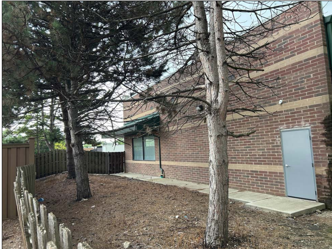
Photo of existing door on east building façade.
