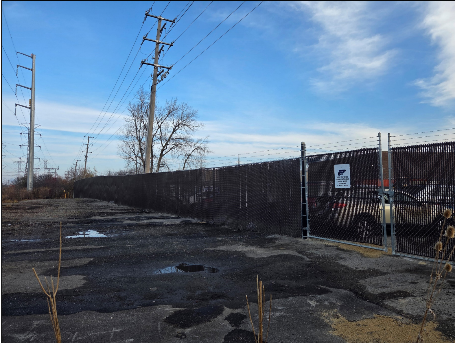
Photo of the new fence on the west property line.
