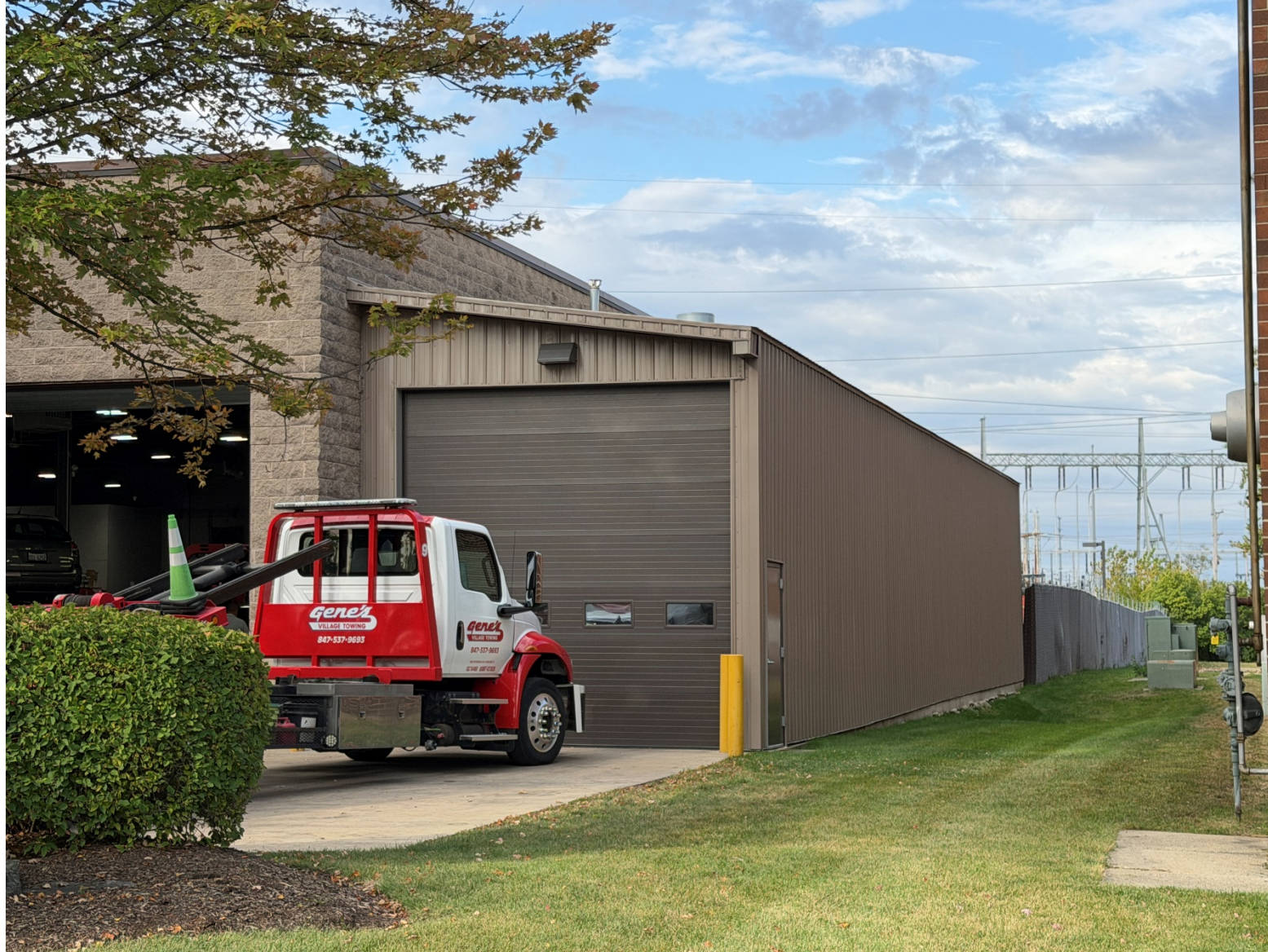
Photo of building addition from Peterson Drive facing West.
