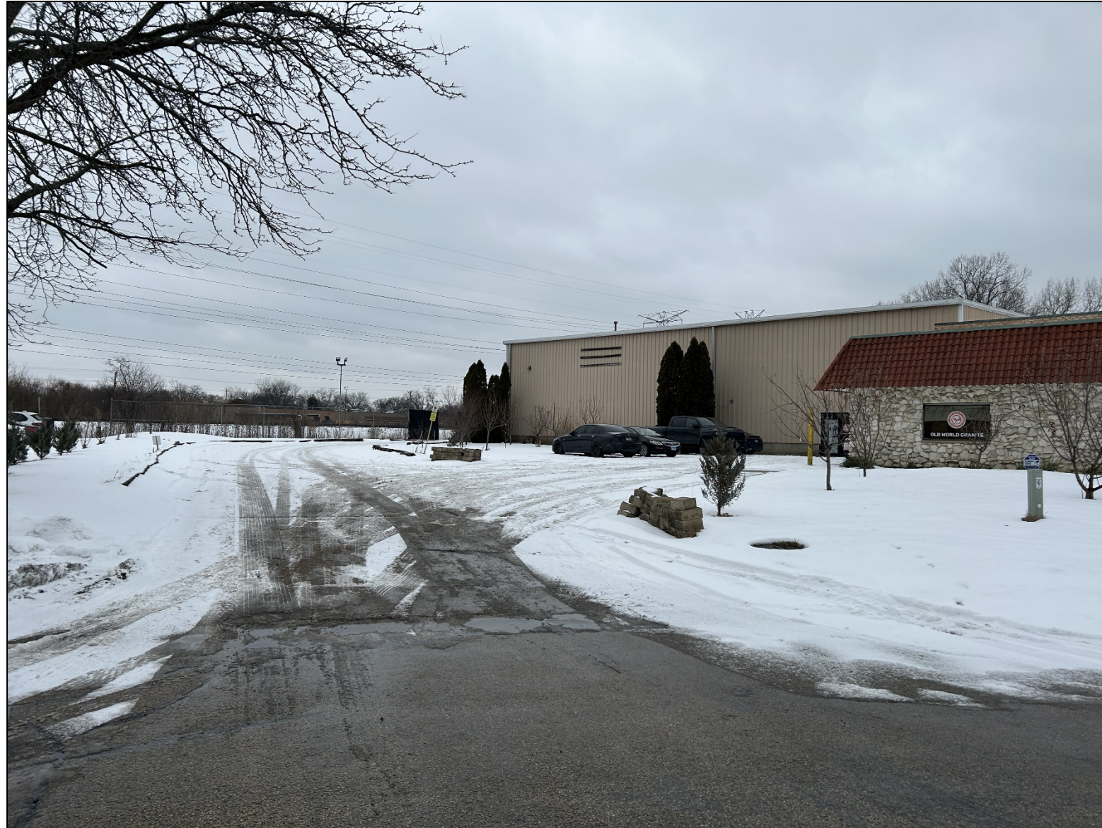
Existing Front of the Building and Driveway West of Building
