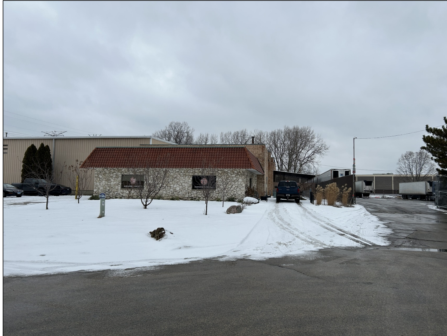
Existing Front of the Building
