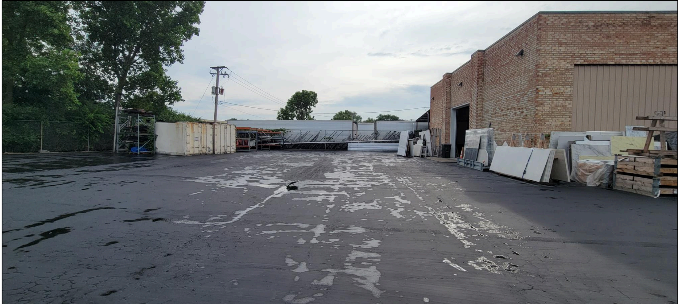
Area Behind Building
