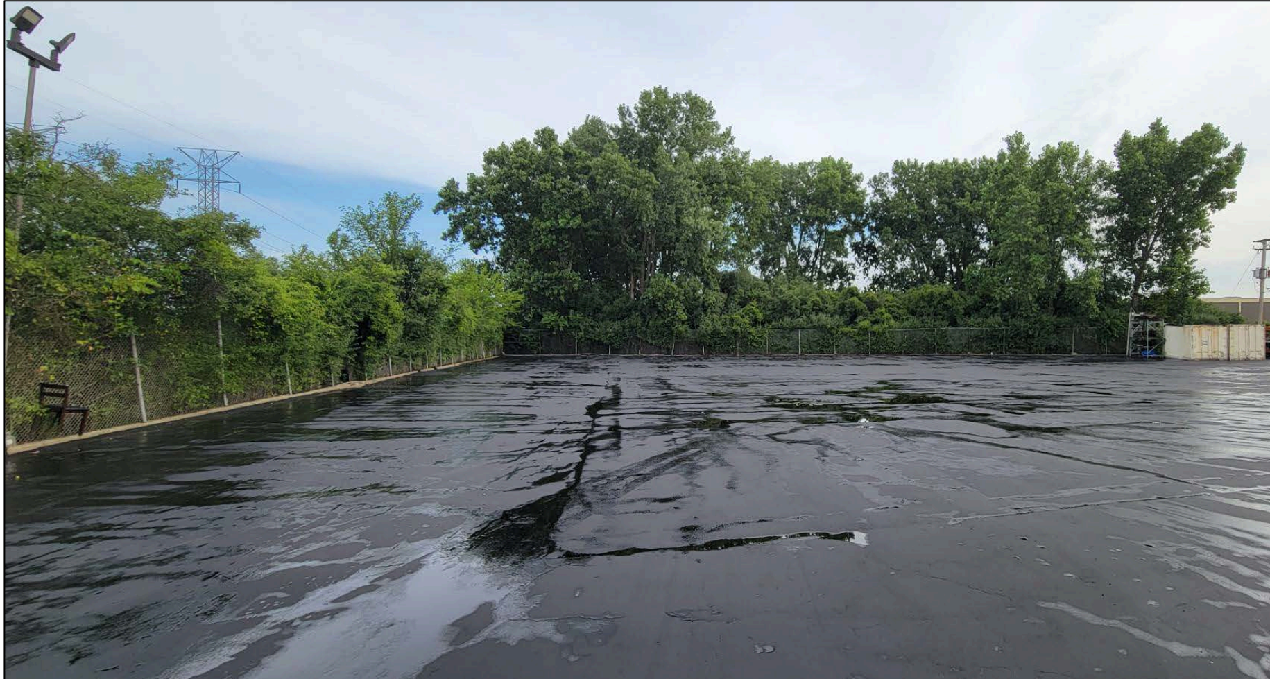
Existing Parking Lot
