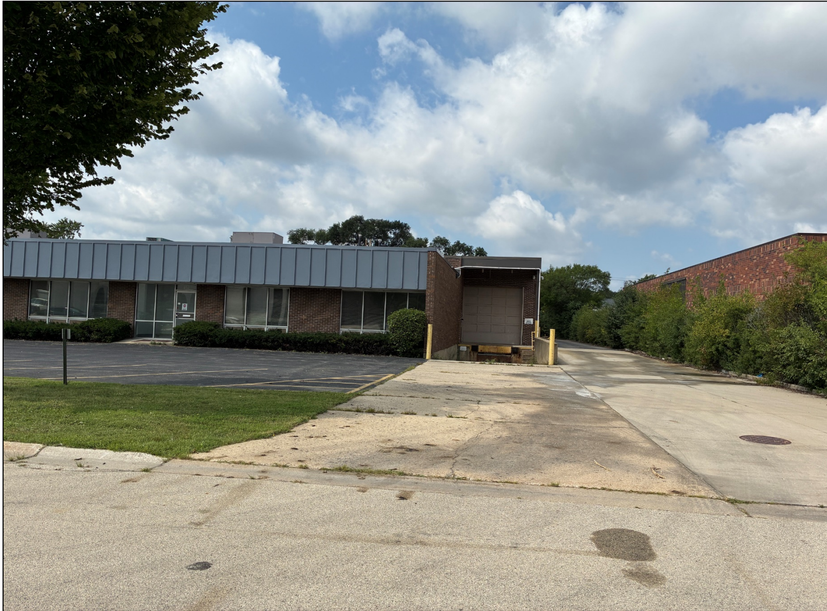
Photo of the north end of the building facing west.
