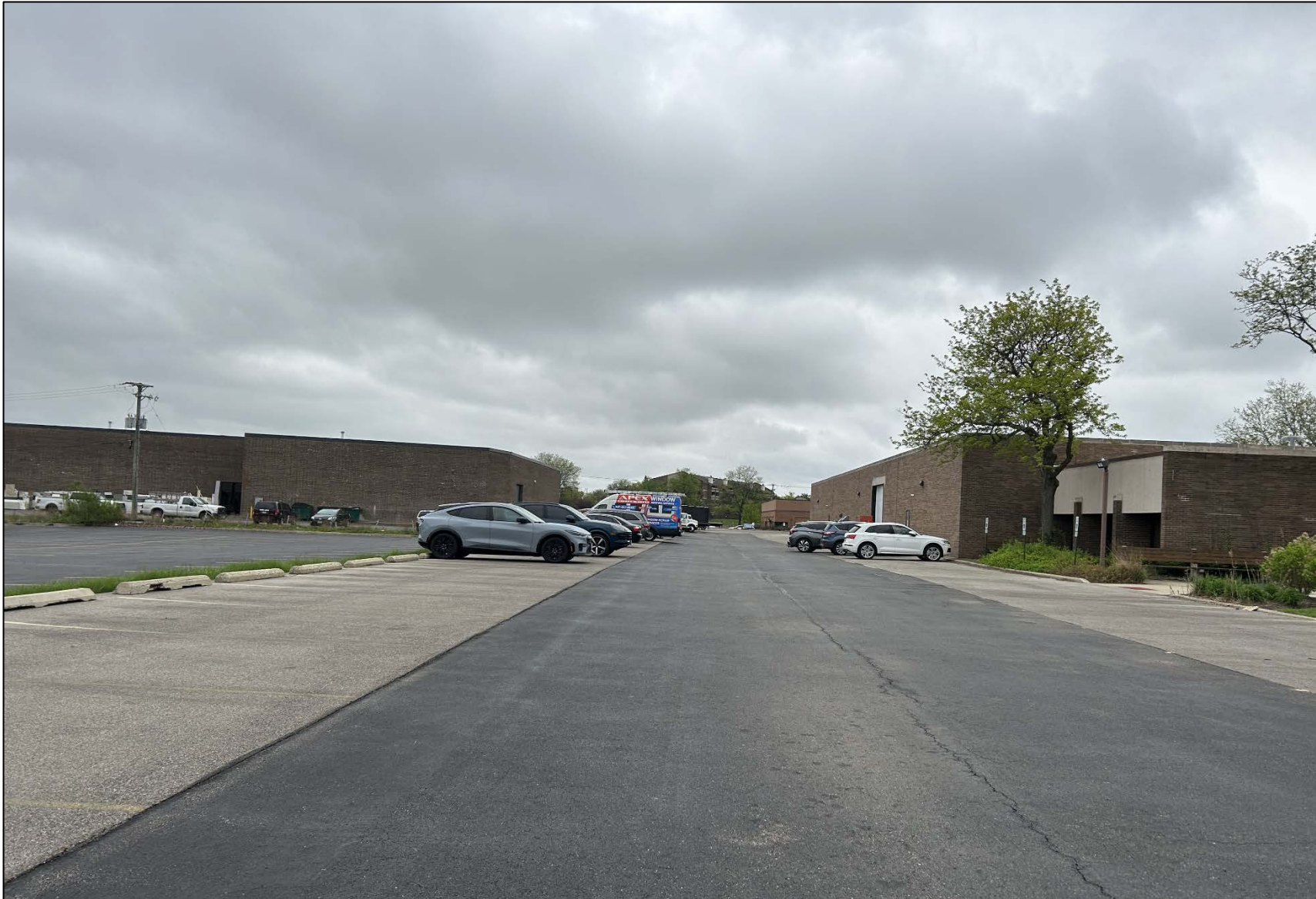
Photo of parking lot on east side of building facing south from Holbrook Dr.
