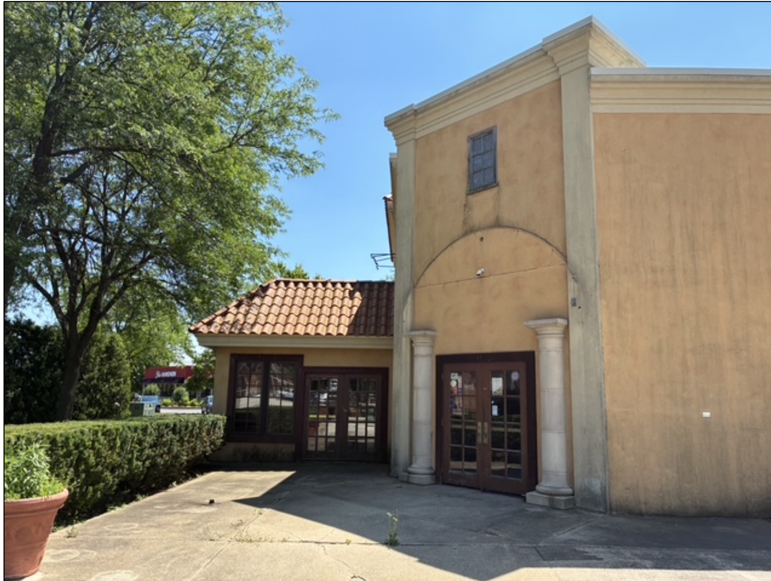
Photo of the front entrance to the building facing south.
