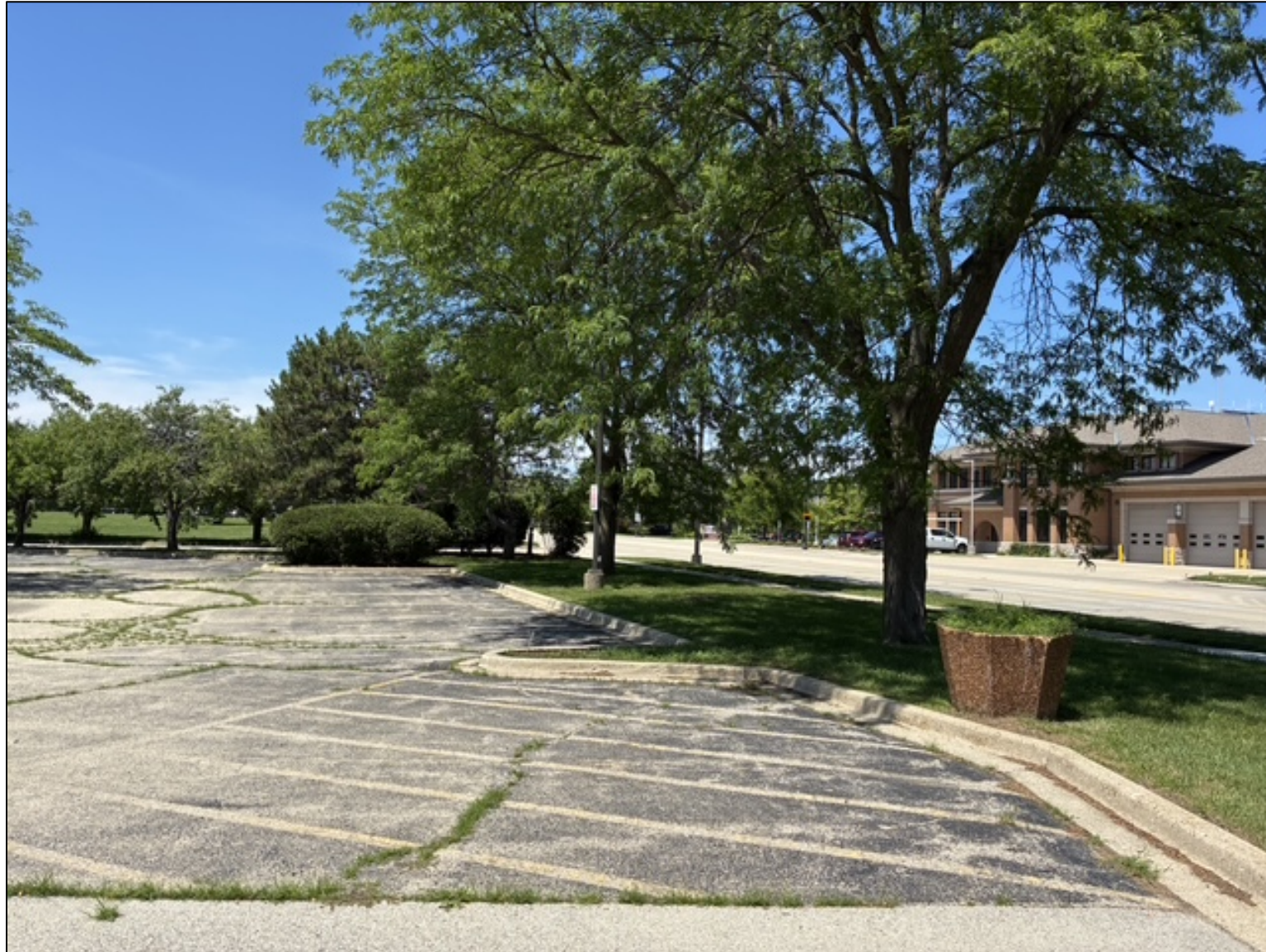
Photo of the parking lot along Milwaukee Avenue facing north.
