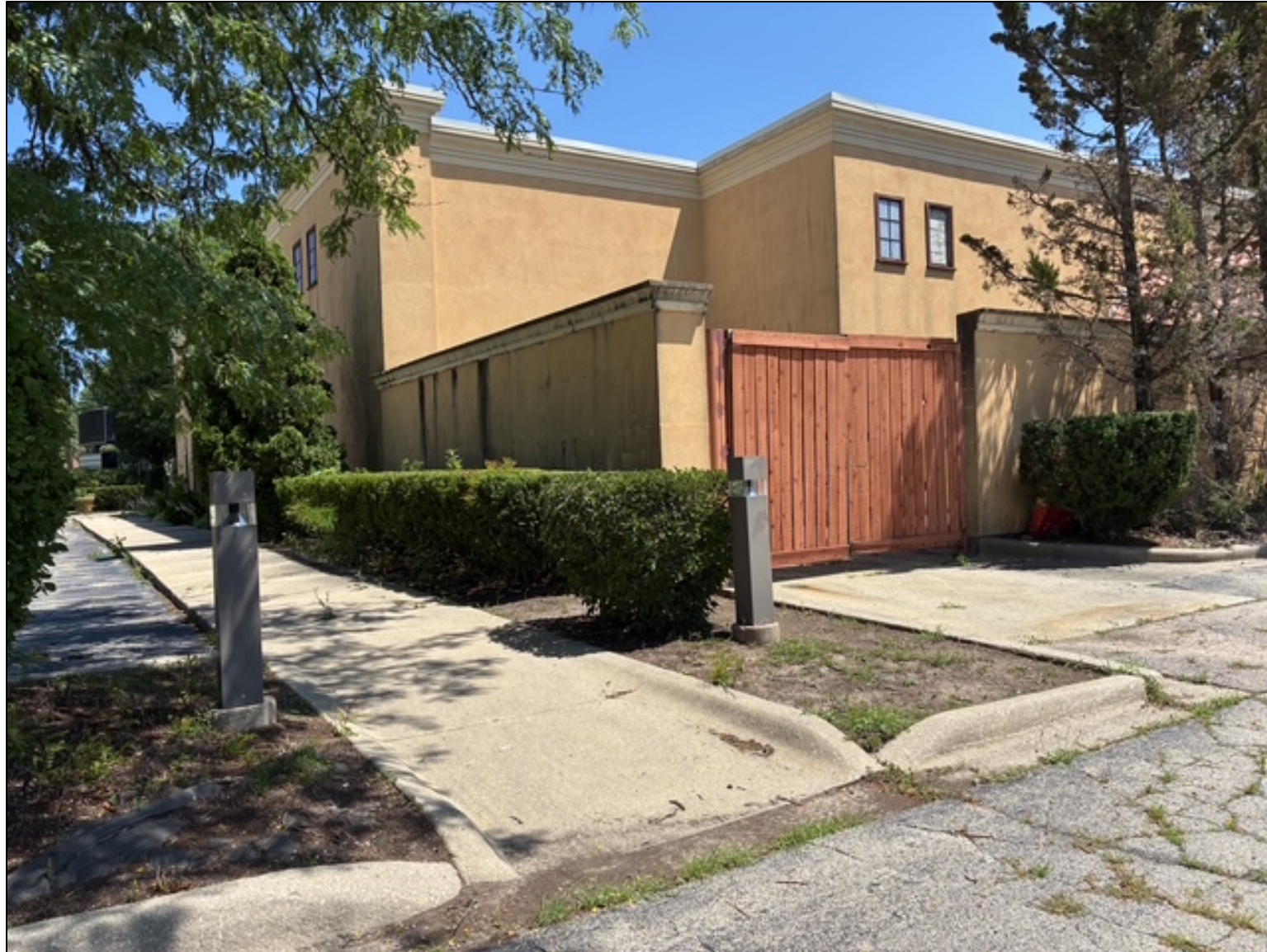
Photo of the trash/utility enclosure on the west side of the building facing east.
