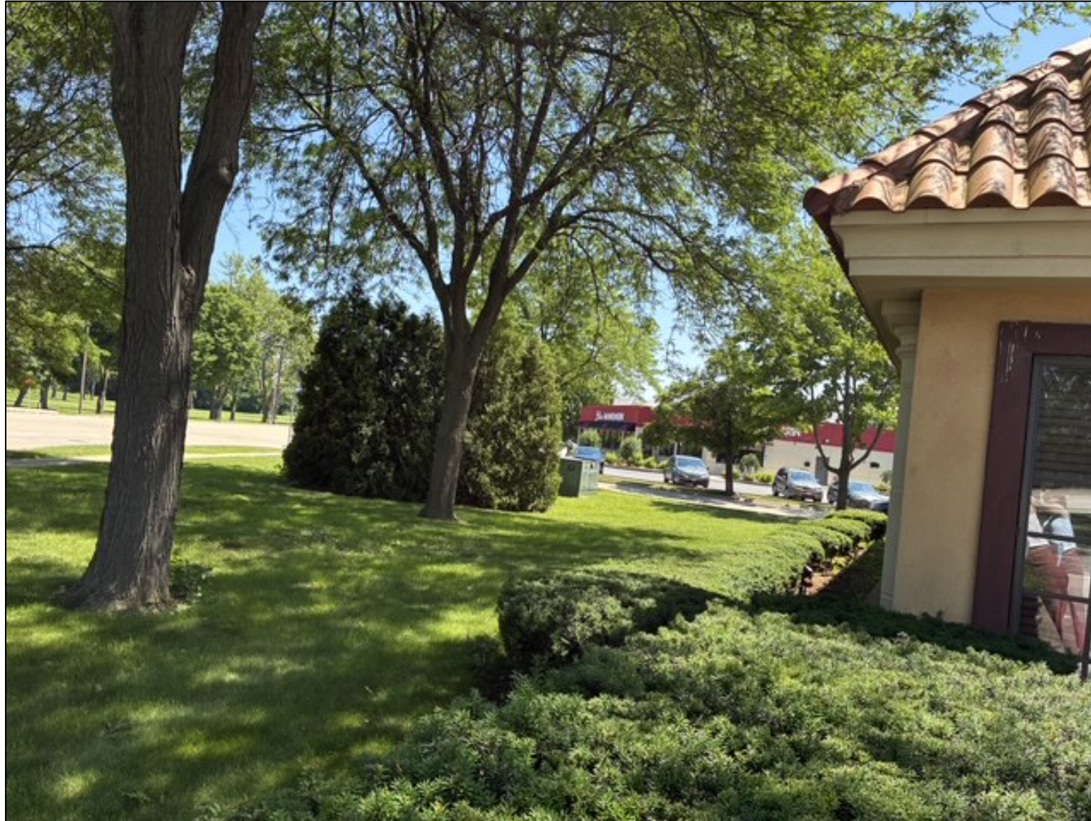
Photo of the area north of the existing building facing south.
